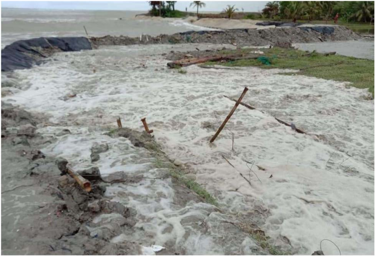
Plate 154 &155– Breached Embankment , Tidal Saline Water Ingression, Sumatinagar , Sagar Block . 21°42'27.11"N 88° 9'16.30"E
