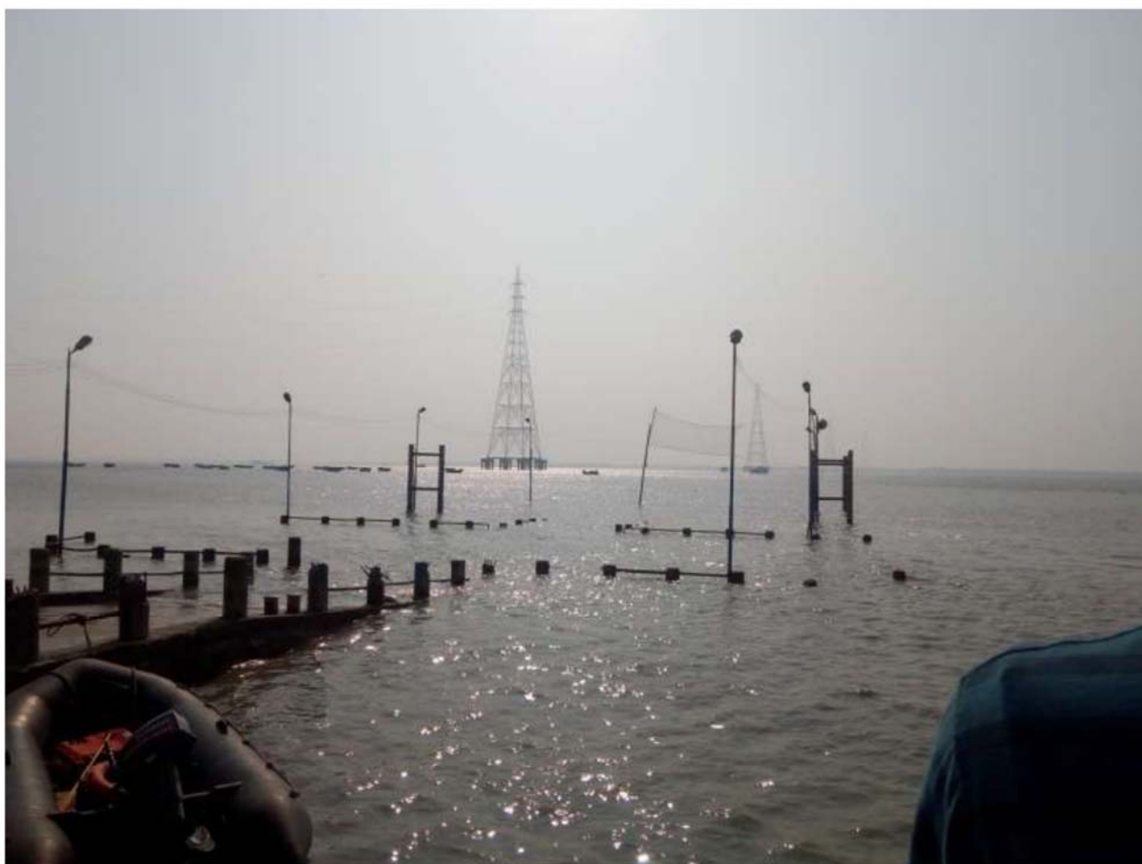
Plate 99– Kakdwip Hardwood Point Jetty , connecting Sagar & Ghoramara Island
