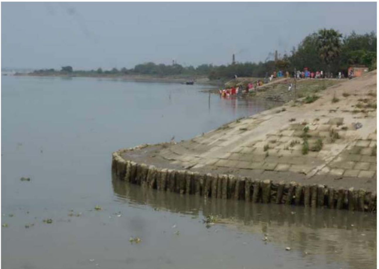
Plate 41– River Hugli near Acra /Akra Ferry Ghat , northern boundary of South 24 Parganas. 22°30'45.55"N 88°12'34.47"E
